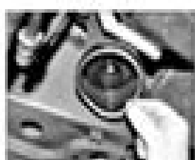
10.31 Fit a new sealing ring to the filter housing.
